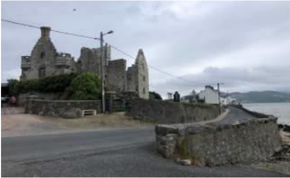
Image 13: Rathmullan Abbey as viewed from the existing slipway off Main Street
