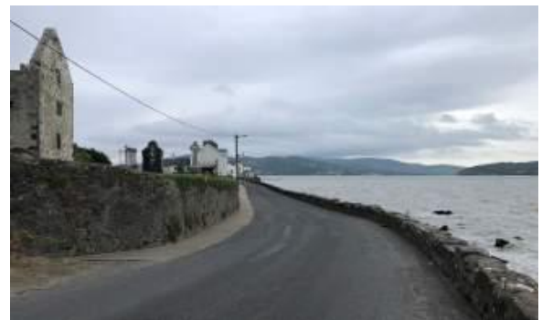
Image 20: Rathmullan Abbey as viewed from the existing slipway off Main Street
